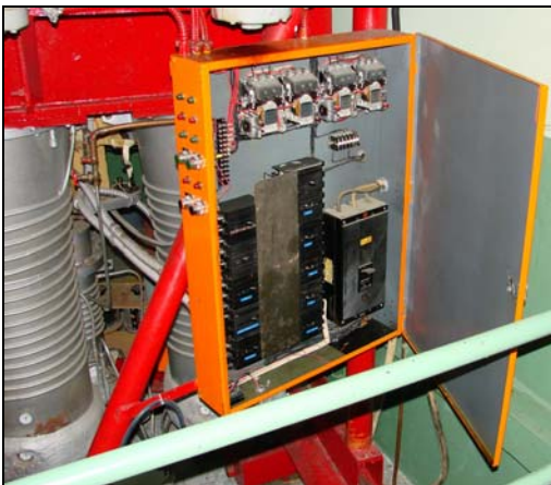
The two bottom breakers are labeled "DIF PUMP 1 & 2"
