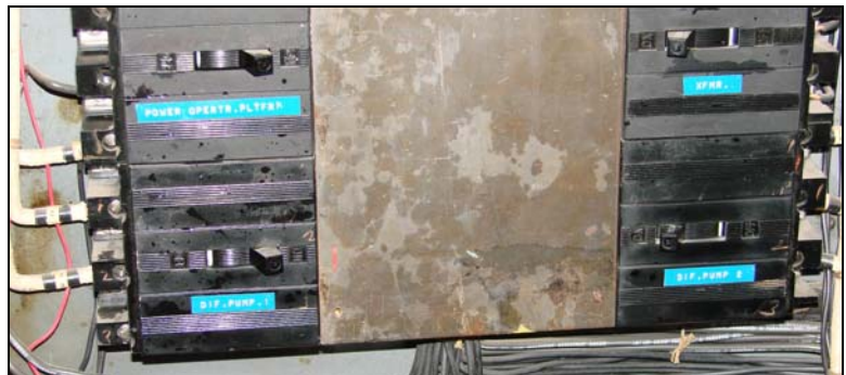
The two bottom breakers are labeled "DIF PUMP 1 & 2"
